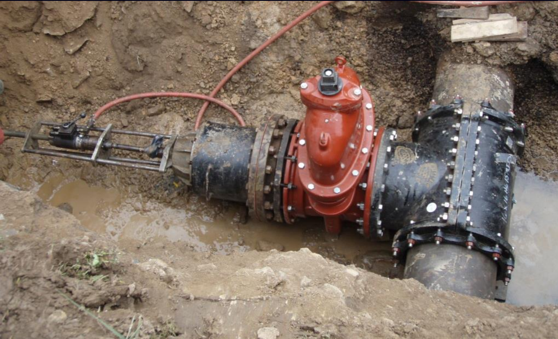
16" x 16" Montgomery Transmission Main Tapping Sleeve & Valve
