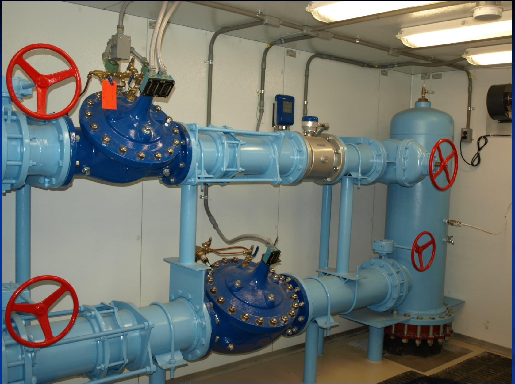
Montgomery Tank Control Valves
