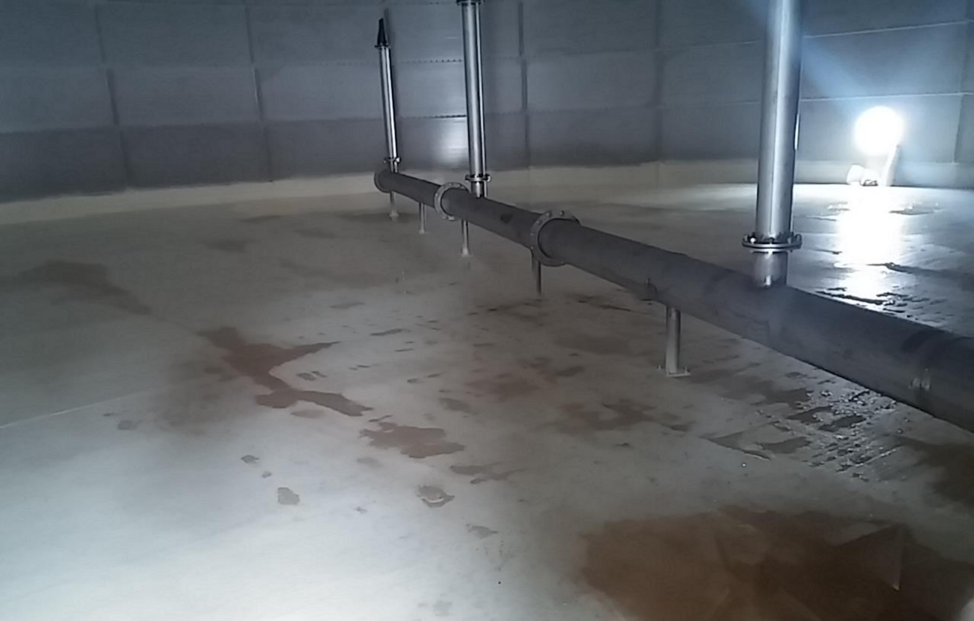
0.5 MG Wolf Run Tank Mixing System
