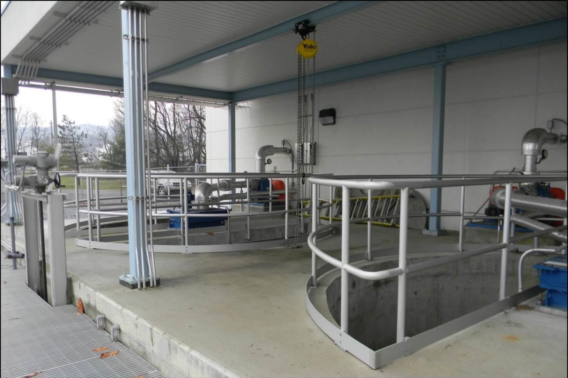
Vortex Grit Separation System (preserve influent carbon)
