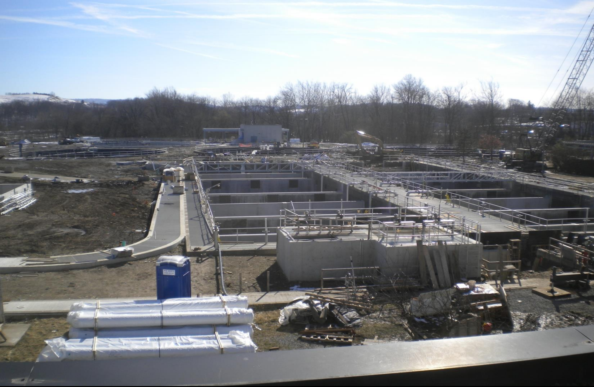
Construction of Aeration Tanks Conversion, Distribution Box and Adjacent Step-Feed Channel
