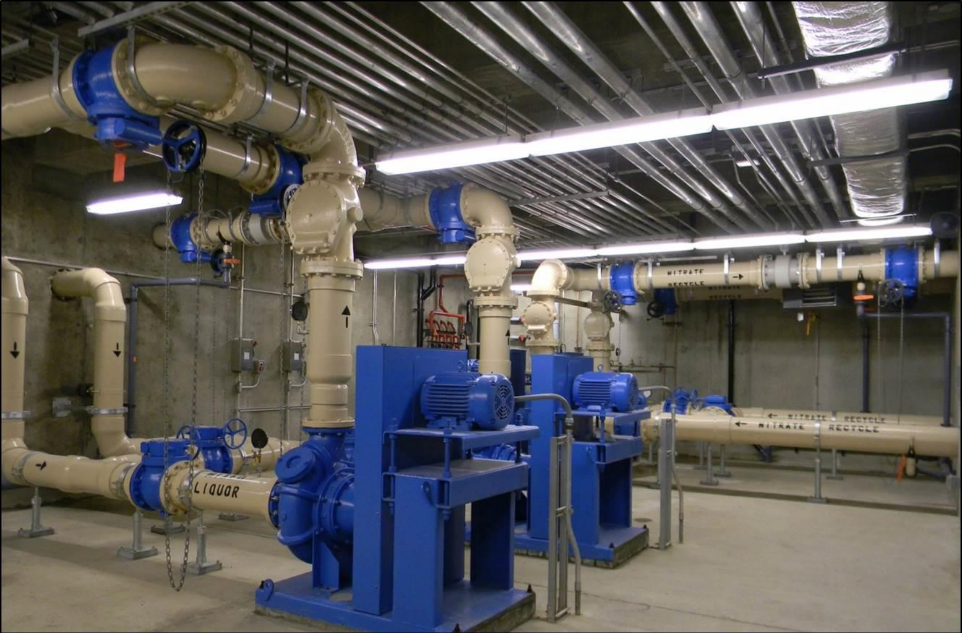
Internal Recycle Pumps – Mixed Liquor & Nitrate
