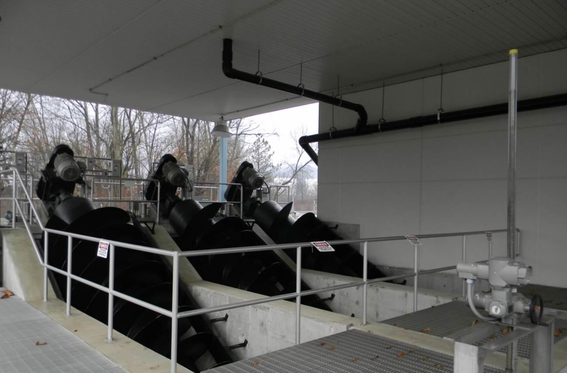
60" Diameter Screw Lift Flood Pumps
