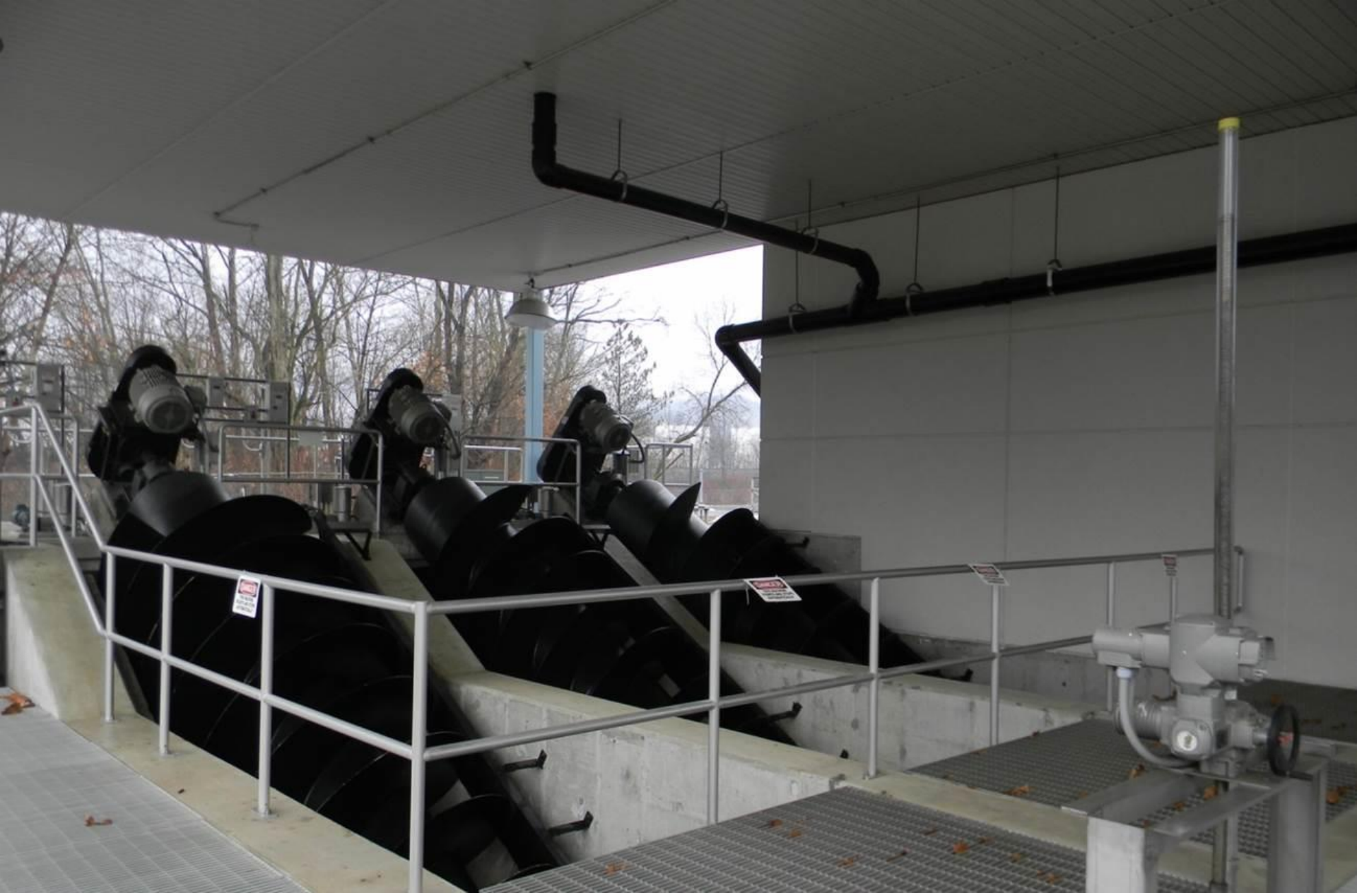
60" Diameter Screw Lift Flood Pumps
