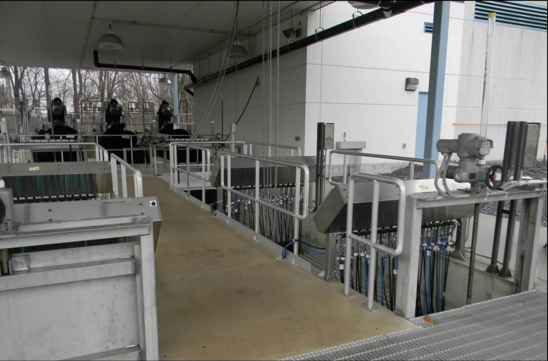
Ultraviolet Disinfection System
