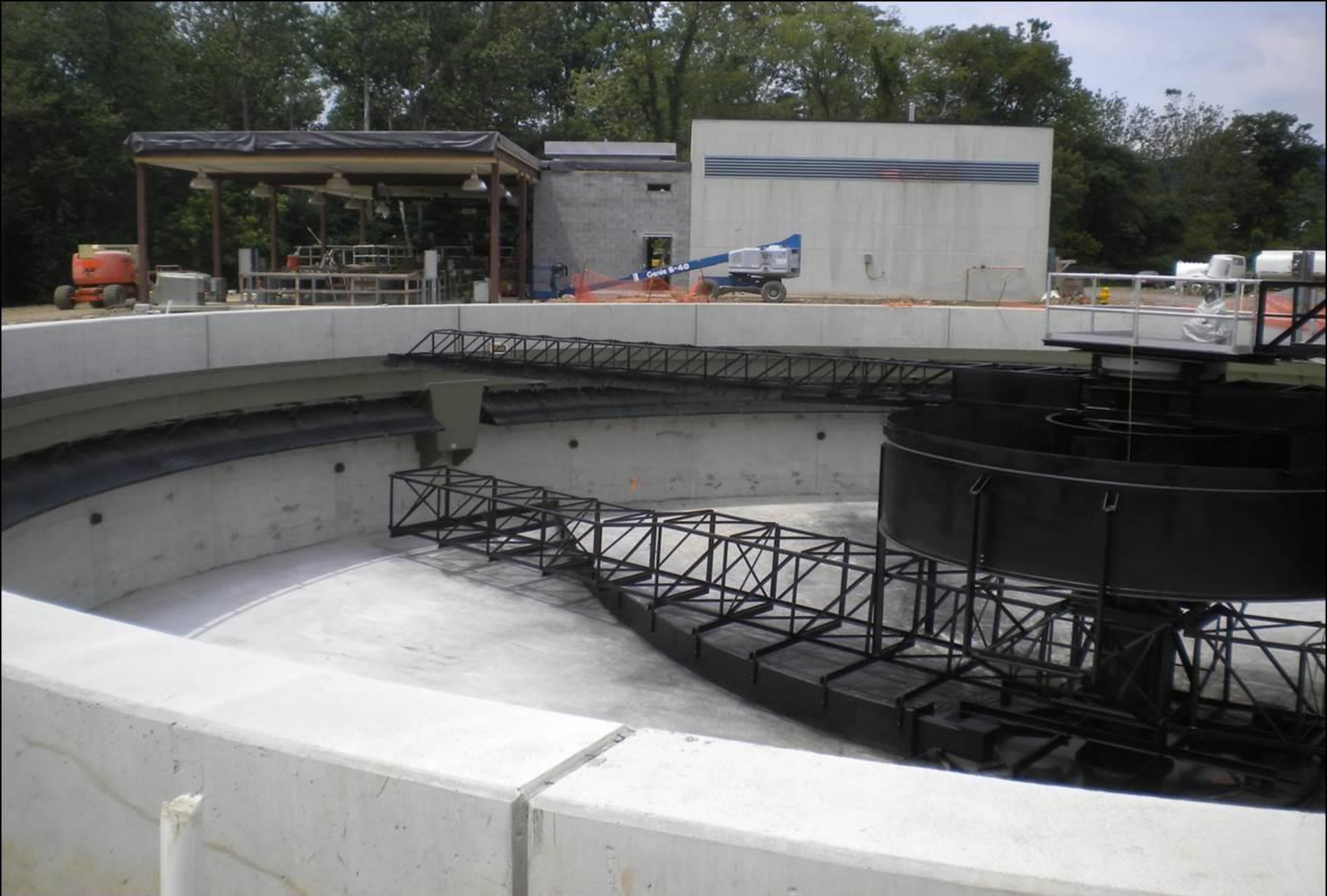
Final Clarifiers with Stamford Baffles
