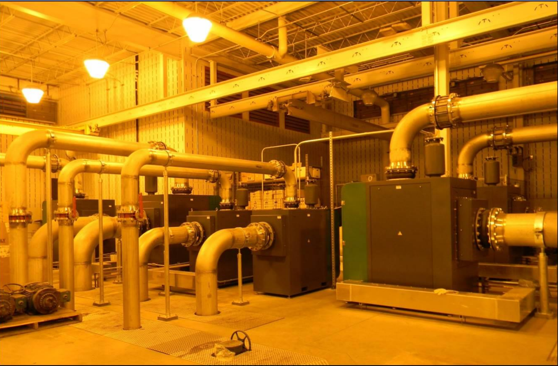
Energy Efficient Turbo Blowers (high turndown capability)
