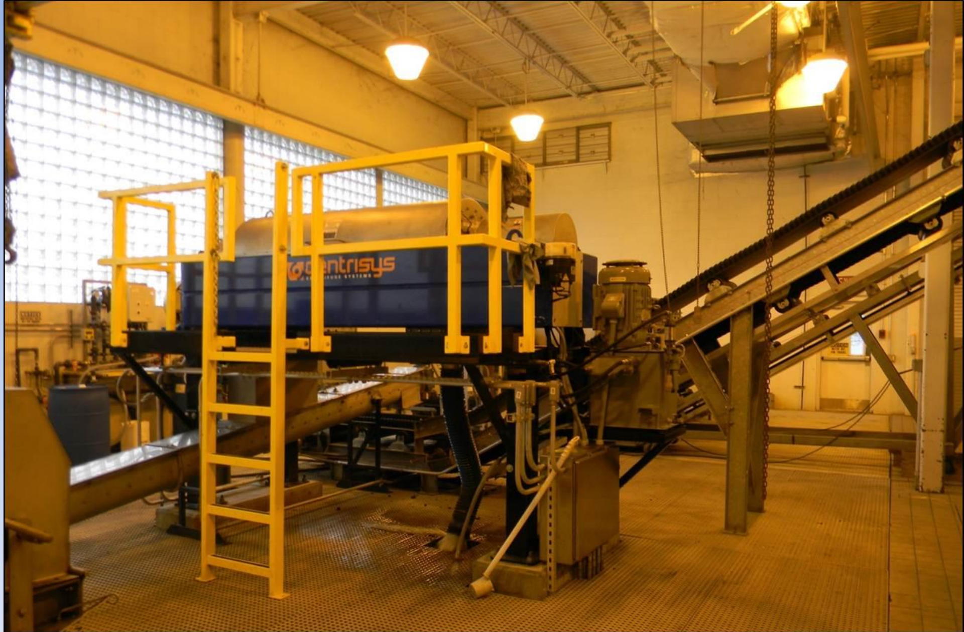
Centrifuge Sludge Dewatering System
