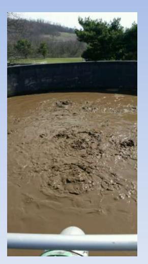
Two Circular Aerobic digesters with a capacity of 691,000 gallons per side. Each side can be operated independently (parallel) or in series. Sludge can be fed to the thickener or the centrifuge.
