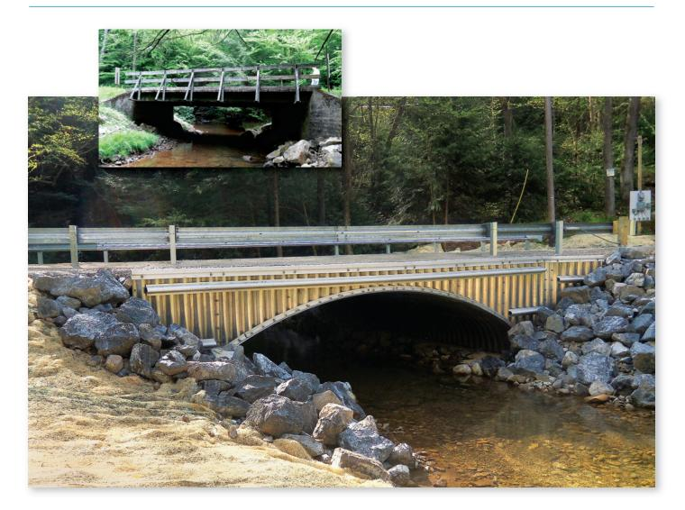
Built in 1948, the JC-16 Bridge was a narrow substandard multi-beam steel stringer bridge with a timber deck. A replacement structure through the conventional PennDOT process would have cost \$750,000.
