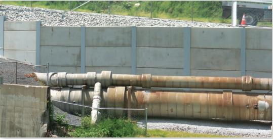
Gwin, Dobson & Foreman designed an earth retaining structure to stabilize a Pittsburgh street next to an existing water treatment plant and large diameter pipelines of the Pennsylvania American Water Company. A unique design provided for a steel H-pile wall and precast concrete lagging panels to replace a failing retaining wall on Madeline Street in the City of Pittsburgh.
