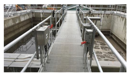
The East Providence Township Municipal Authority selected Gwin, Dobson & Foreman, its long time consulting engineer, to design the replacement of its process treatment system. An Intermittent Cycle Extended Aeration System (ICEAS) was selected as the biological treatment process with nutrient removal capability.
