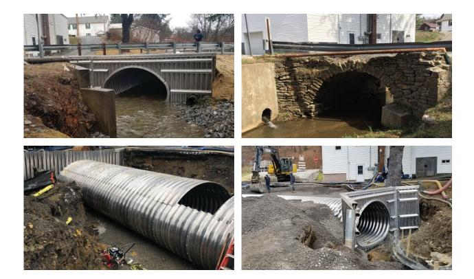
Gwin, Dobson & Foreman served as the design engineer for the replacement of a deteriorating concrete and stone arch bridge on Spruce Street (T-459), which spans an unnamed tributary to Elk Run. GD&F designed a cost-effective solution using an aluminum structural plate pipe-arch structure with aluminum wing walls.
