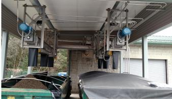
The Pennsylvania-American Water Company planned a new solids handling system at its Clarion Wastewater Treatment Plant. PAWC chose Gwin, Dobson & Foreman to provide a complete, engineered solution for the dewatering, conveying and storing of residual waste solids from the treatment process.
