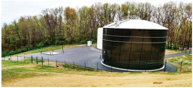
The Pennsylvania-American Water Company contracted Gwin, Dobson & Foreman to design a new water storage tank and access road to its McHenry Hill tank site in Indiana, PA. The project included the construction of a 750,000-gallon, glass-lined bolted steel storage tank; Overlook Drive access road and site improvements, 20-in. fill and draw water mains; stormwater management; tank drain facilities; control valve vault and instrumentation and control system.
