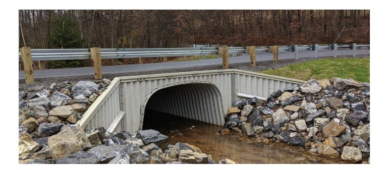
Gwin, Dobson & Foreman served as the design engineer for the replacement of a deteriorating concrete bridge on Clearfield Street (T-862) in Cooper Township, which spans an unnamed tributary to Moshannon Creek. GD&F designed a cost-effective solution using an aluminum structural plate pipe-arch structure with aluminum wing walls and full invert bottom.
