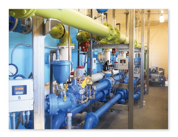
Gwin, Dobson & Foreman designed improvements to the Dallas State Correctional Institution's water supply and treatment system. The project involved a comprehensive hydrogeological analysis of the existing well waters, replacement of the 1980's era filtration system and improvements to the instrumentation and control system. Major work elements included:
