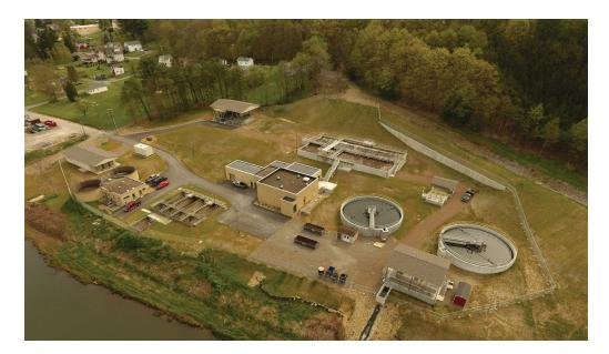
In response to a PA DEP consent order to eliminate sewer overflows and plant bypassing, the Brookville Municipal Authority directed Gwin, Dobson & Foreman to provide a solution. After an extensive flow monitoring program and planning study, GD&F recommended that all wet-weather sewer flow be conveyed to the treatment plant. This involved the construction of a wet-weather pumping station, new interceptor sewer system and upgrade and expansion of the wastewater treatment plant.
