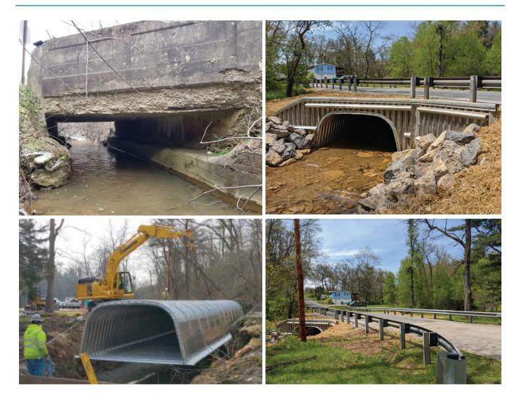
Gwin, Dobson & Foreman designed the replacement of a 100-year old concrete bridge on Black Road in Elk Township which spans an unnamed tributary to Deer Creek. GD&F's design is a cost-effective solution using an aluminum structural-plate box culvert with aluminum wing walls and full invert bottom.
