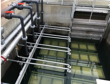
Gwin, Dobson & Foreman designed a membrane bioreactor replacement system that provides enhanced wastewater treatment and process operation at the Tuscawilla WWTP. GD&F performed an assessment of the membrane bioreactor (MBR) system operations and recommended a more compatible and efficient membrane filtration system.
