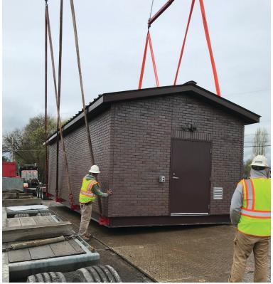
Gwin, Dobson & Foreman designed a new water booster station for the Montandon area of the Pennsylvania-American Water Company - Milton District. The station replaced an existing pumping facility that had reached the end of its useful life. Three new booster pumps were installed, each with a capacity of 500 gpm.
