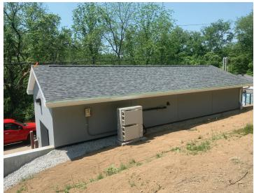
Gwin, Dobson & Foreman designed a new water booster station for the Mill Hill area of the Pennsylvania-American Water Company – Mon-Valley District. The station replaced an existing pumping facility that had reached the end of its useful life. Three new booster pumps were installed, each with a capacity of 750 gpm.
